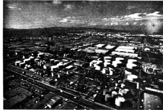
Powerine Oil Company's modern high conversion refinery in Santa Fe Springs.
